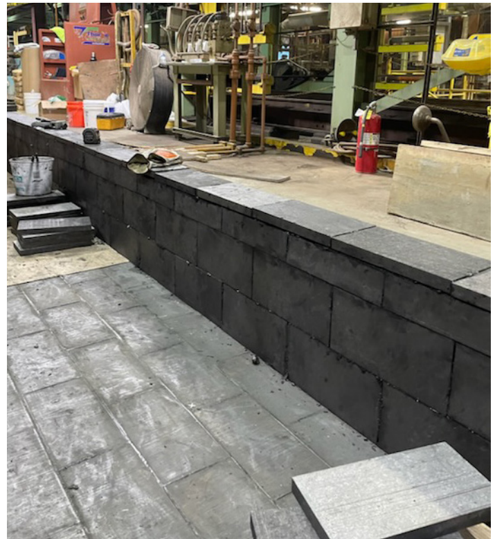
Tile Installation – Graphite tile on floor and curbing
